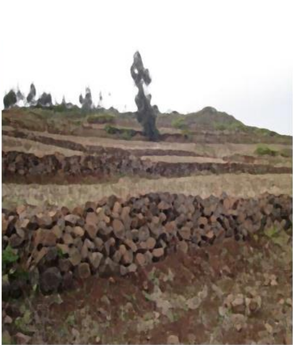
Stone bunds / aligning stones along 1m.contours - in slopes steeper than 1:10, and in the parts not covered with vegetation.
